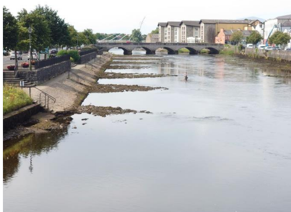
Sites M3/4 Cathedral Pool with boulder deflectors visible at low tide on the Cathedral Road side – salmon migration route / fishing area (22 July 2021)
