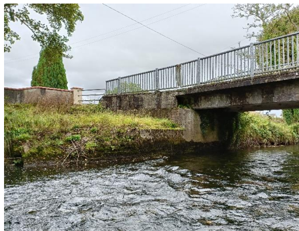
BR3a – Brusna/Glenree: Shanaghy Heights Bridge – bank and bed protection extending 6m downstream (11 September 2023)
