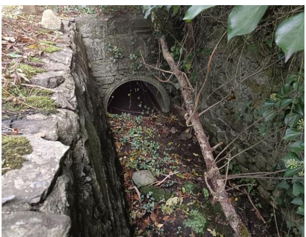
QG5 – Quignamanger, dry culvert ("diversion culvert" to be replaced) upstream of the flowing stream emerging from the flap valve (11 Sept. 2023)
