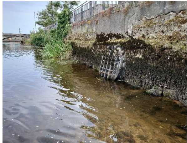
Site M9/10 Existing river walls on Ridgepool RHS and non-return culvert flap (22 July 2021)
