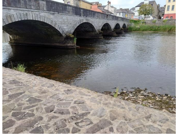
Site M5/6 Cathedral Pool - Existing bank defences and instream habitat with deflectors (low tide) (22 July 2021)
