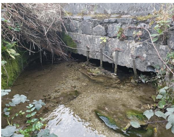
QG5 – Quignamanger, existing culvert beneath Quay Road (to be replaced with correctly sized box culvert) (11 Sept. 2023)
